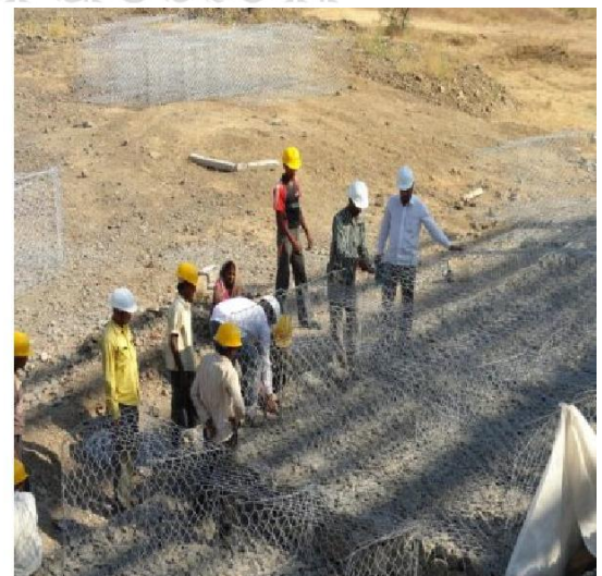
Fig:05 Placing of empty gabion boxes
