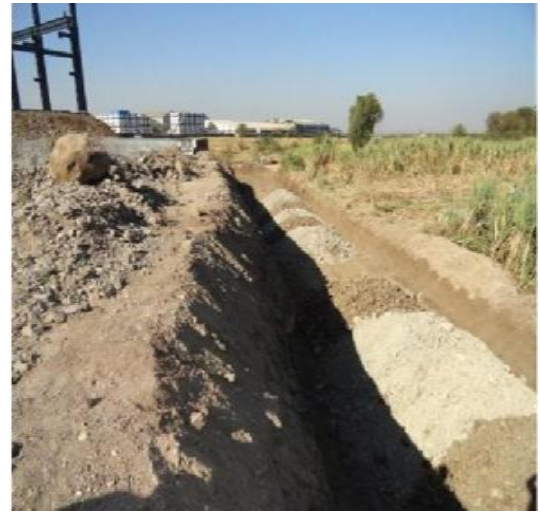
Fig:03 Soil Replacement
